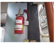
Automatic fire extinguisher system of the electrical cabinet
